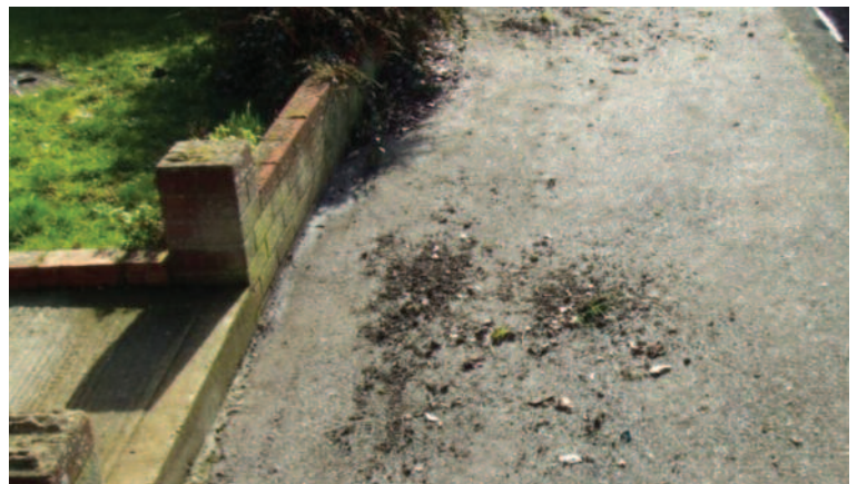
Detritus builds up along edges of footways and kerbs and where weeds will take hold. In this photo, mechanical weed brushing has shifted detritus to the centre and must be cleared
