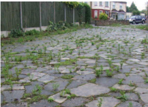
Crazy paving, in pavement planting and cracks in paving all make weed control more difficult
