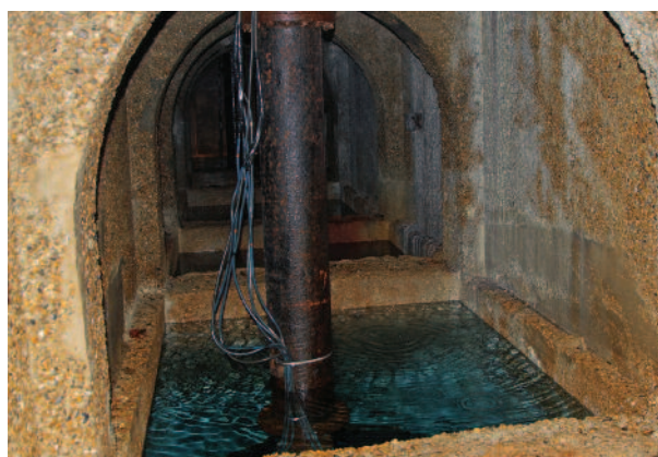
Borehole (Photo: South East Water Ltd.)
