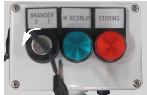
Fig. 5-6: Switch off (1)
